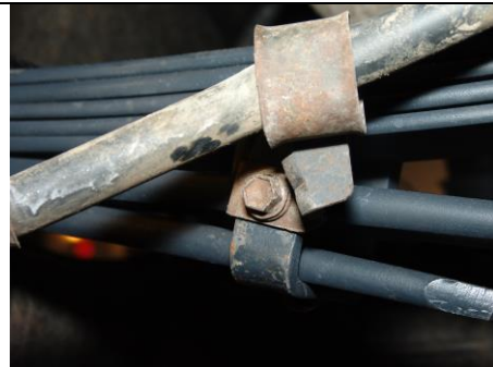
Park Brake cable installed (Step 25)
