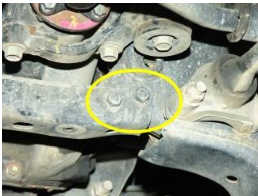
Side bolts of the existing cross member (Step 3B)
