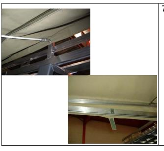
7. Locate fibreglass rod onto M8 bolt and outer awning tube. Push up the rod and close velcro flap to hold rod in place.
